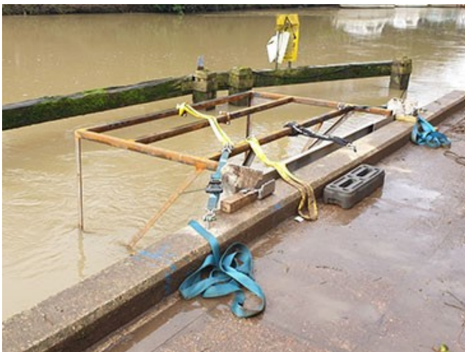
Fixing Frame and Measuring Frame in position
