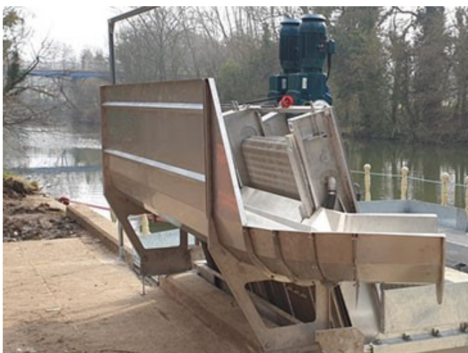
Fitting the Debris Trough and return channel
