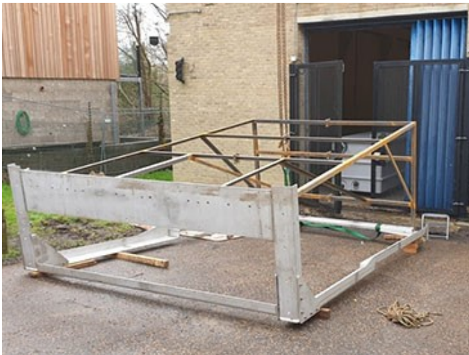
Fixing Frame and Measuring Frame being assembled
