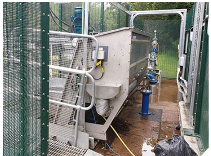
The completed installation, inside the security fencing
