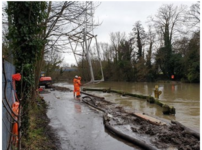
Fixing Frame and Measuring Frame being lifted into the intake – note the very high water levels!
