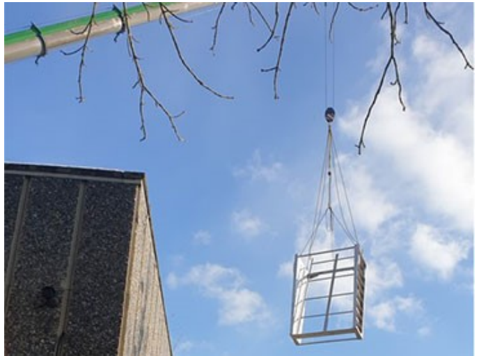
Lifting the assembled Intake Box into the intake with a 60-tonne crane
