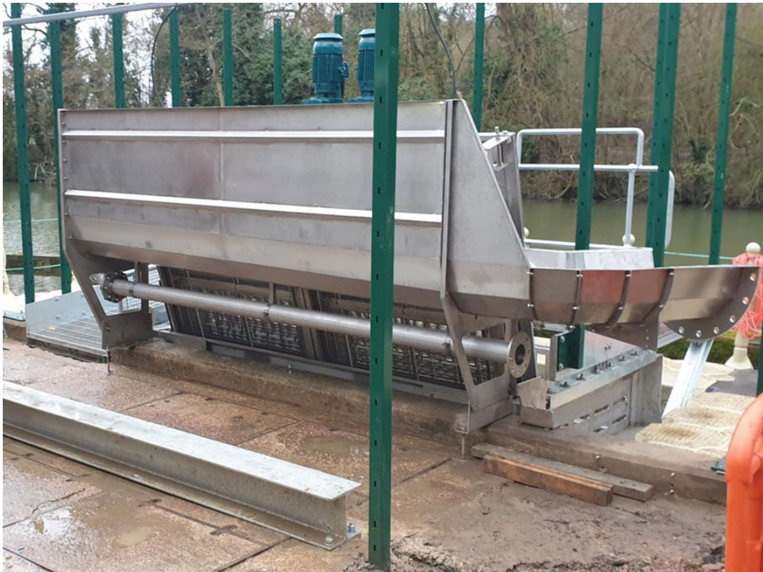
Security fencing being fitted
