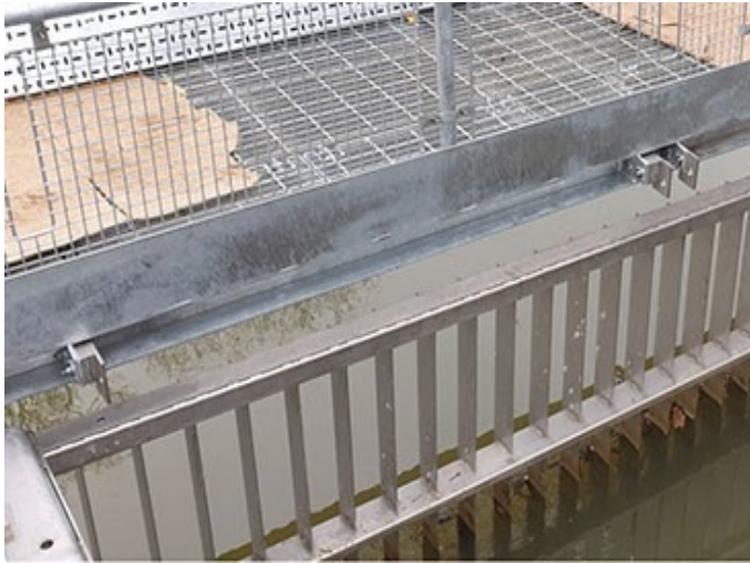
View from the-screens, looking out towards the river
