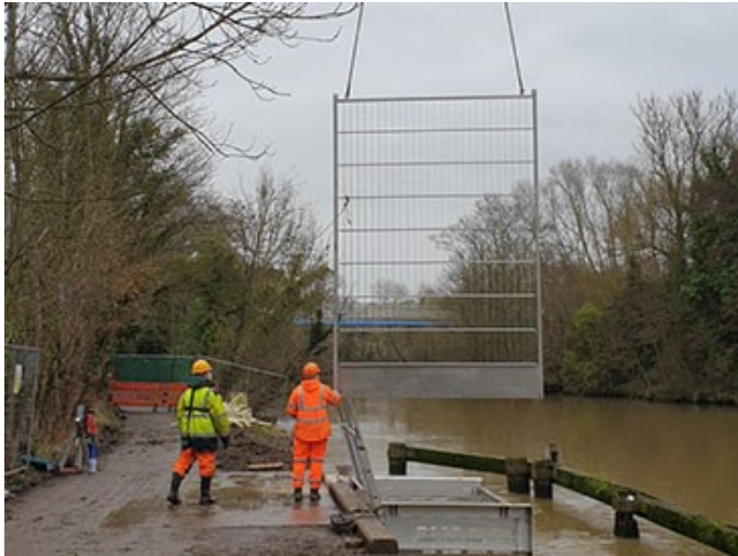
Lifting the course bar screen into the Intake Box
