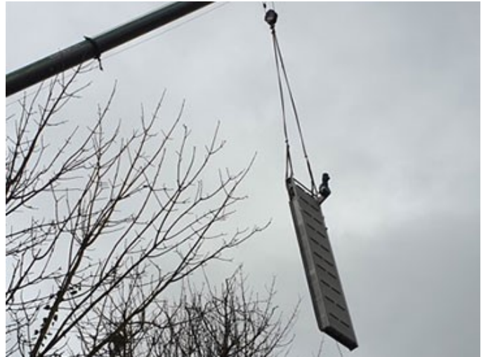
Lifting the first GoFlo screen into the Intake Box
