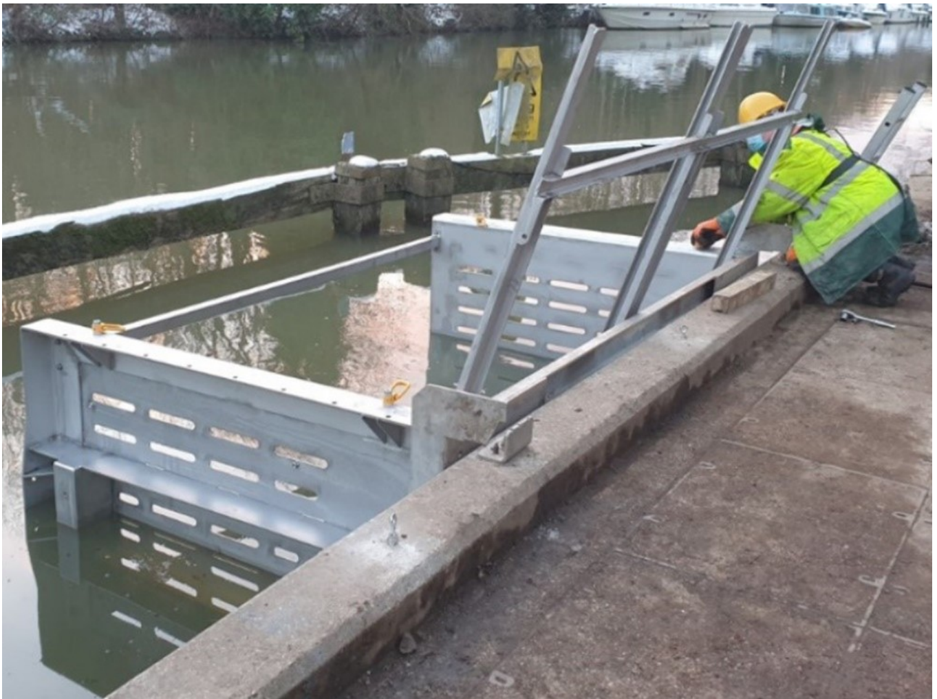
The assembled Intake Box attached to the concrete structure.
