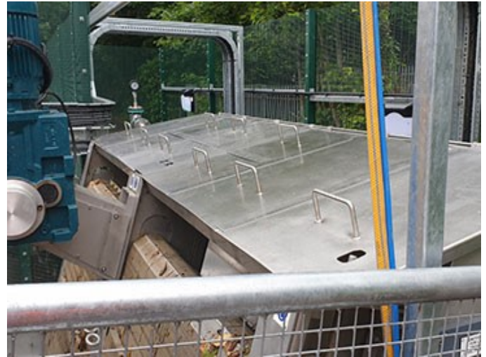
The lids covering the debris trough
