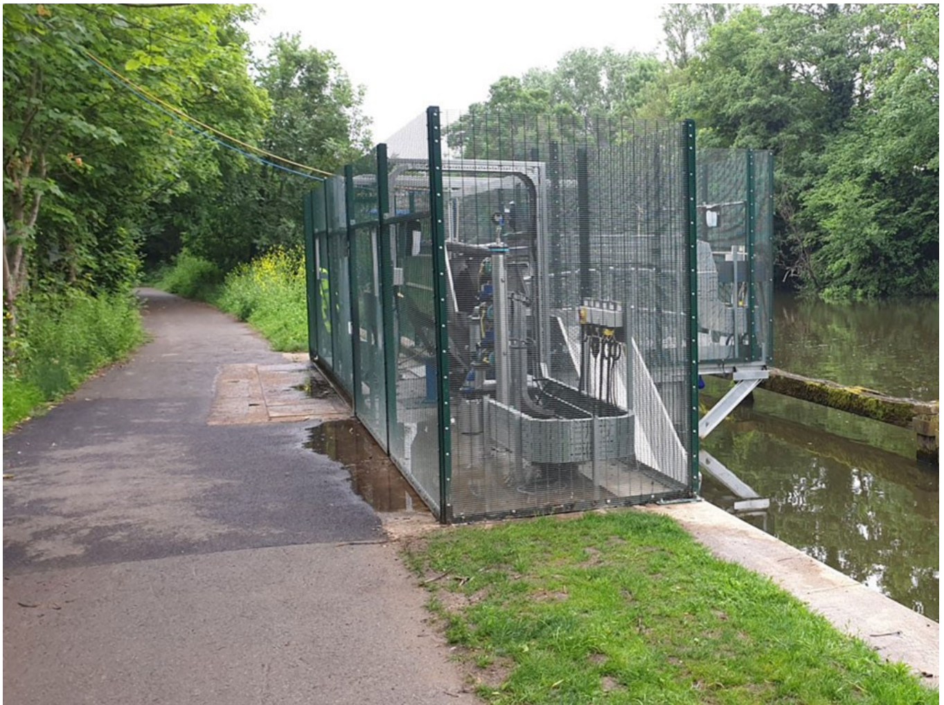
The completed installation, looking upstream
