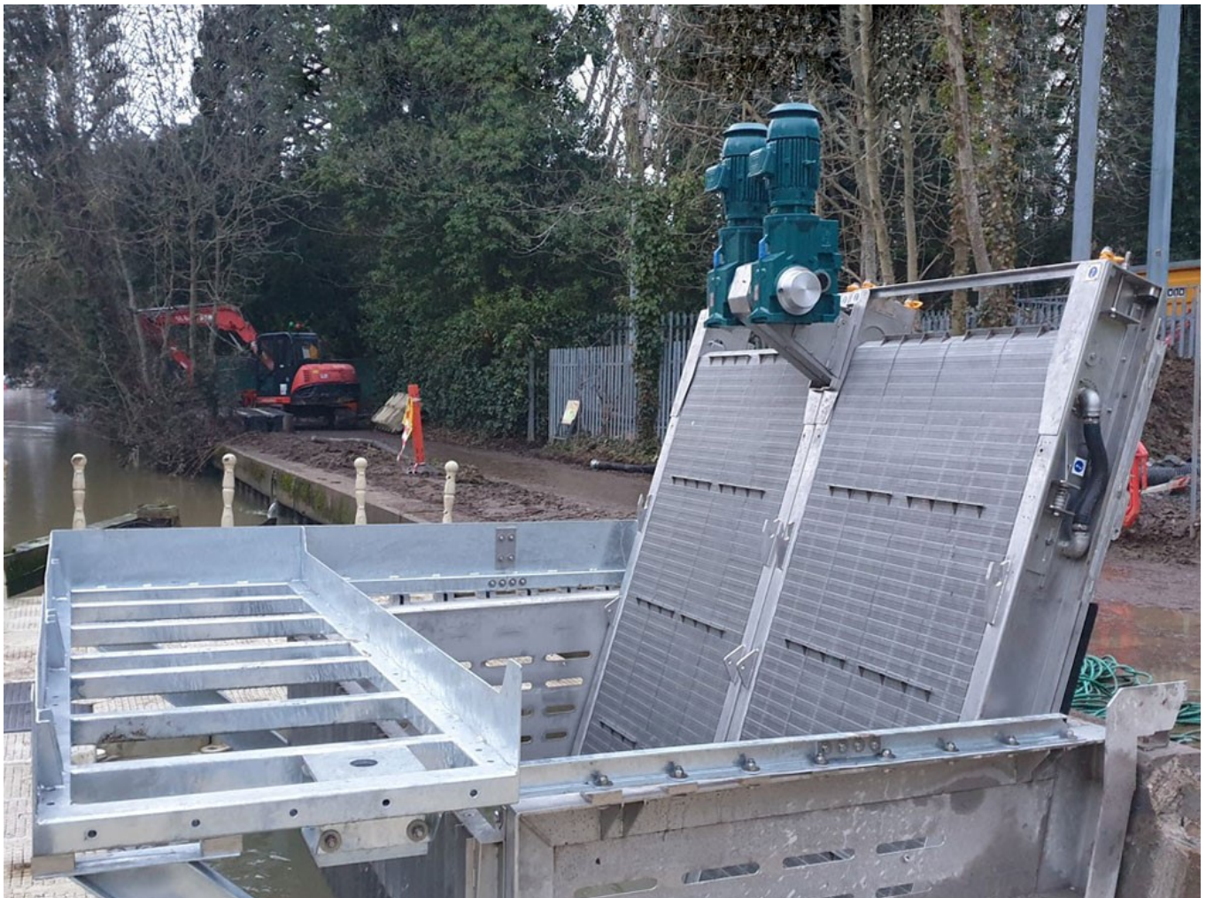
Fitting the front part of the walkway structure onto the Intake Box
