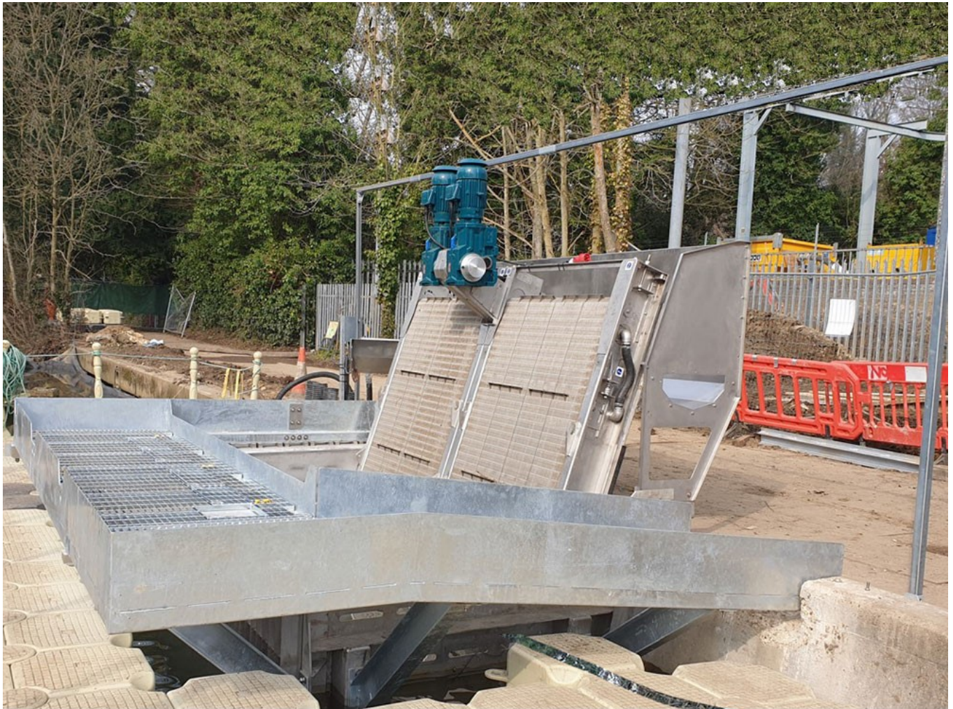
Completed walkway structure attached to the Intake Box
